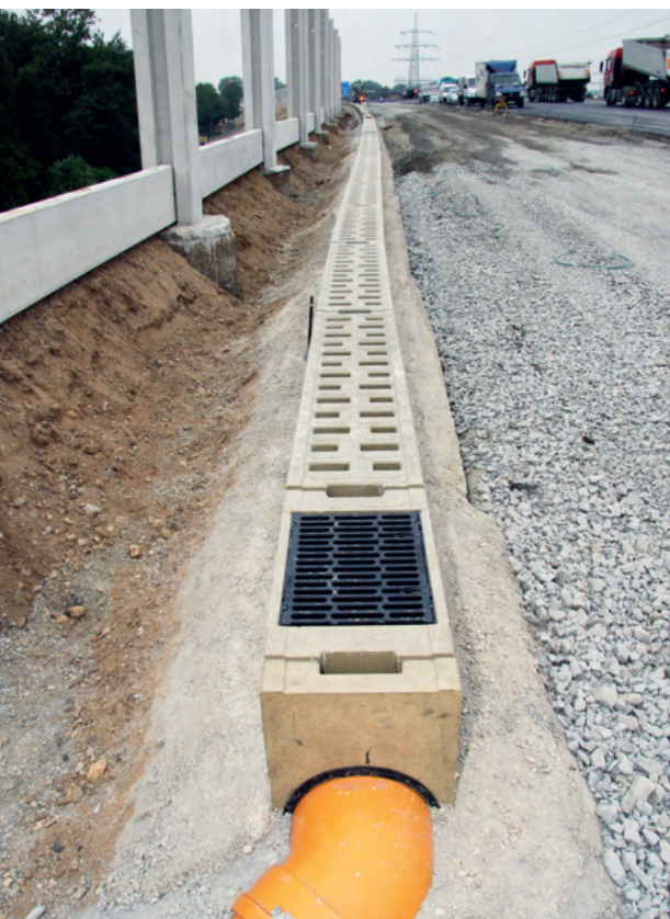
ACO DRAIN® Monoblock RD 300 installation.
